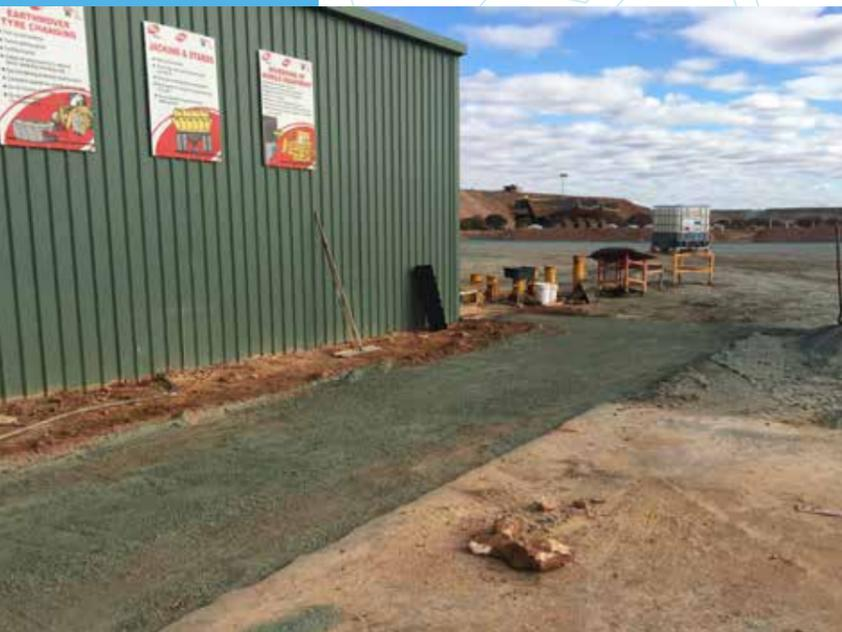
Geohex needs to sit flush with the surrounding ground level, so ensure that final finishing levels have been established during the excavation stage.
